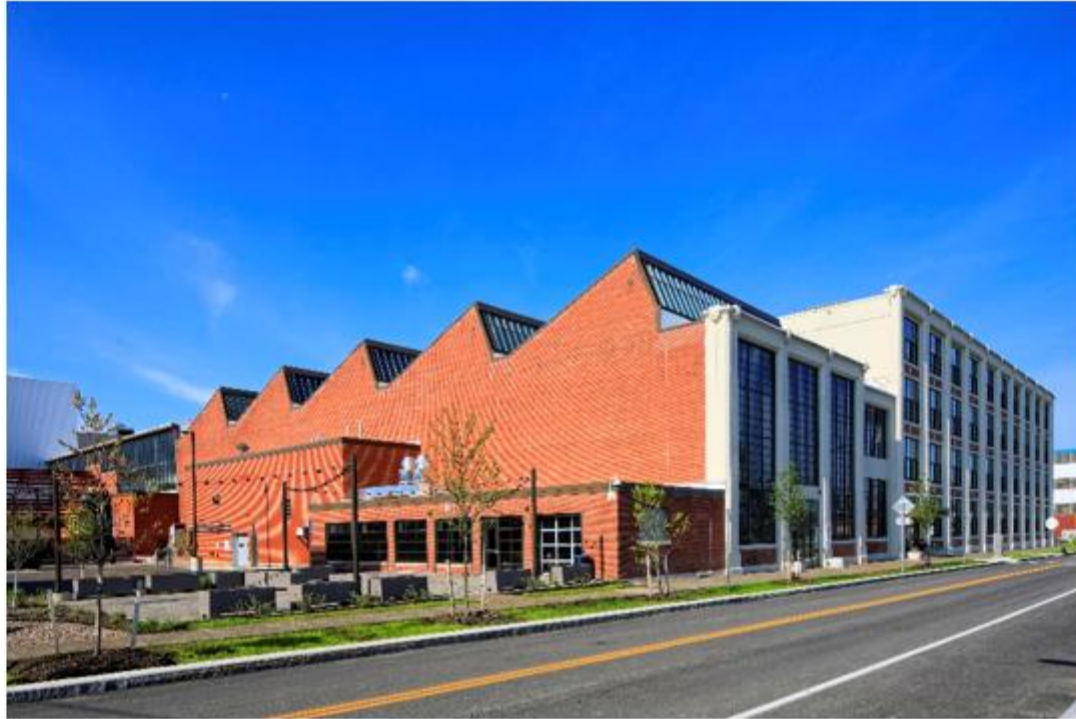
Northland Beltline Neighborhood Redevelopment, Buffalo, NY (Watts)
