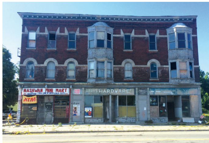
The Ferry Street Hardware Building was torn down by the City of Buffalo in 2018 after being left open to the elements and experiencing significant deterioration by an owner who was unable to care for it.
